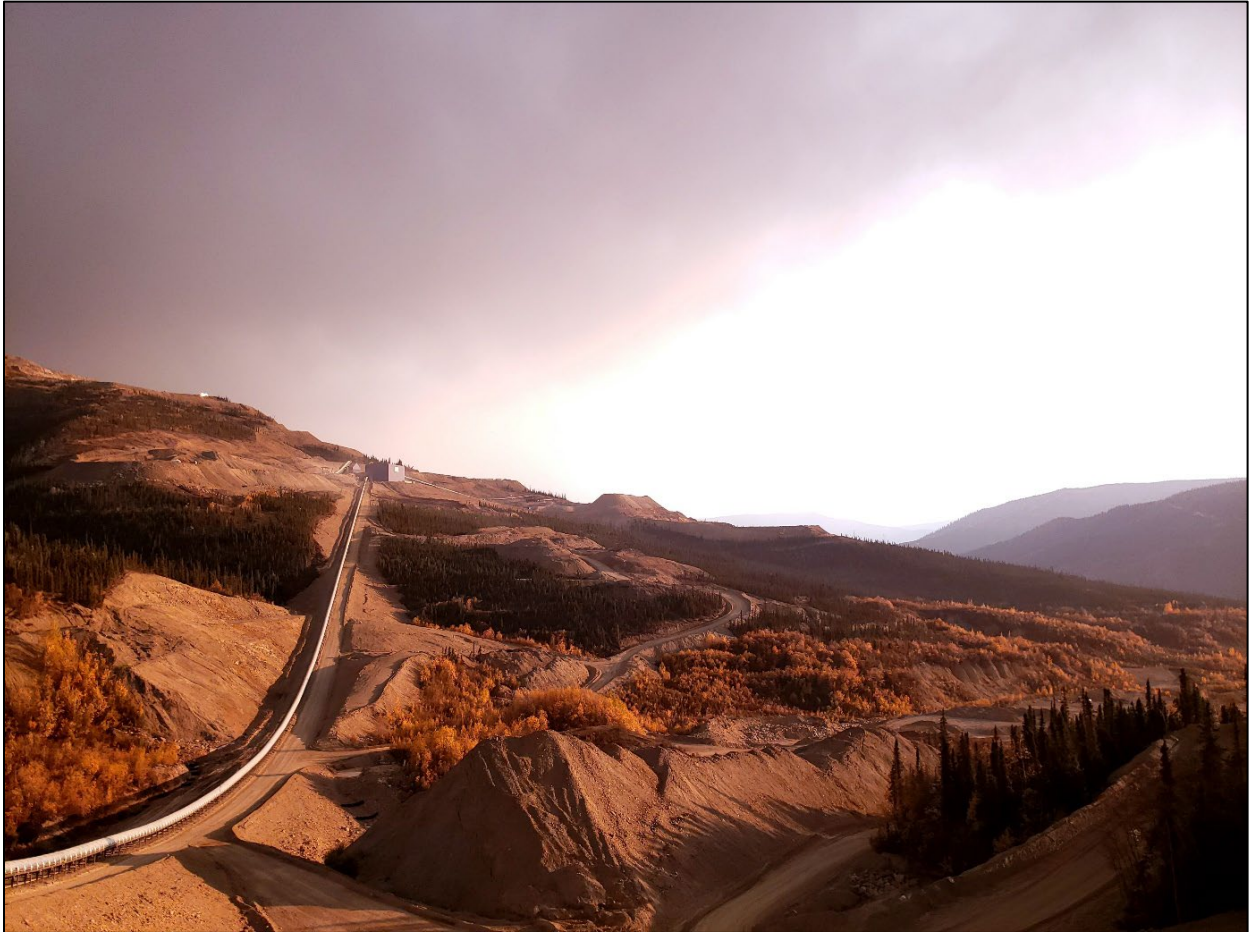
Figure 5-2: Typical Landscape in the Project Area - From primary Heap Leach Facility Facing South Toward Crushing Area and Eagle Pit
