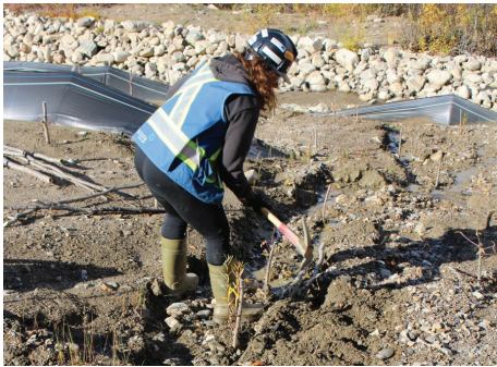
/ Willow staking/pole drain repair (Photo: Kate Hale)
