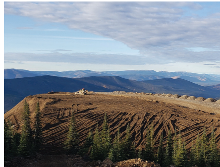
/ Platinum Gulch Pilot scale cover trial overview during construction
