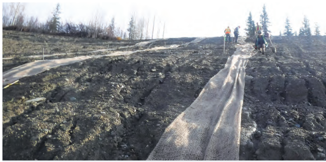
Control pond jute fibre installation and seeding at the Eagle Gold Mine in 2019.
