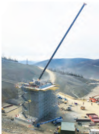
Primary Crusher under construction.
