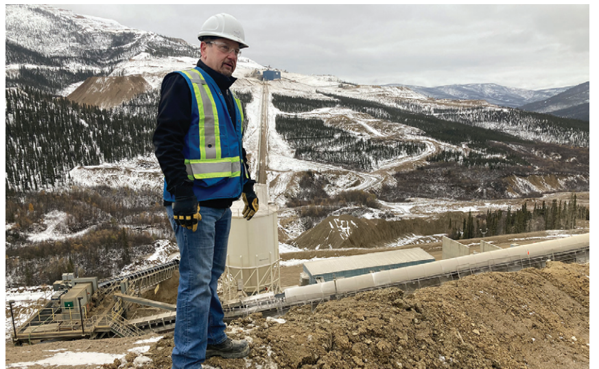
Victoria Gold’s Vice President/Eagle Gold Mine General Manager Kelly Parker overseeing operations at the mine’s heap leach, with a view of the overland conveyor and Secondary/Tertiary Crusher in the background.
