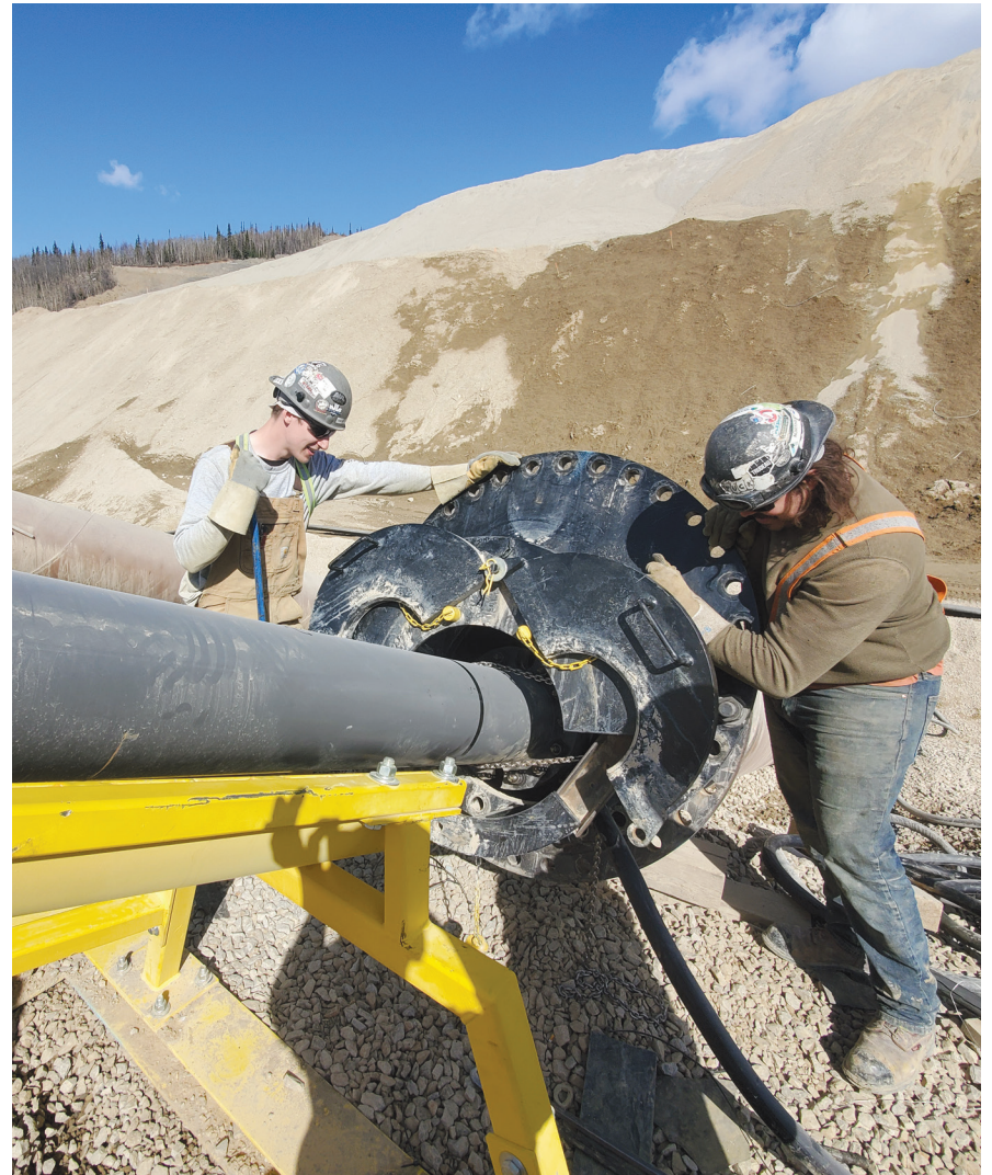
The Eagle Gold Mine's Fixed Maintenance Team, which now includes Cody Joe, shown removing the pregnant solution pump to clean and de-scale and reinstall as part of the site's maintenance program.
