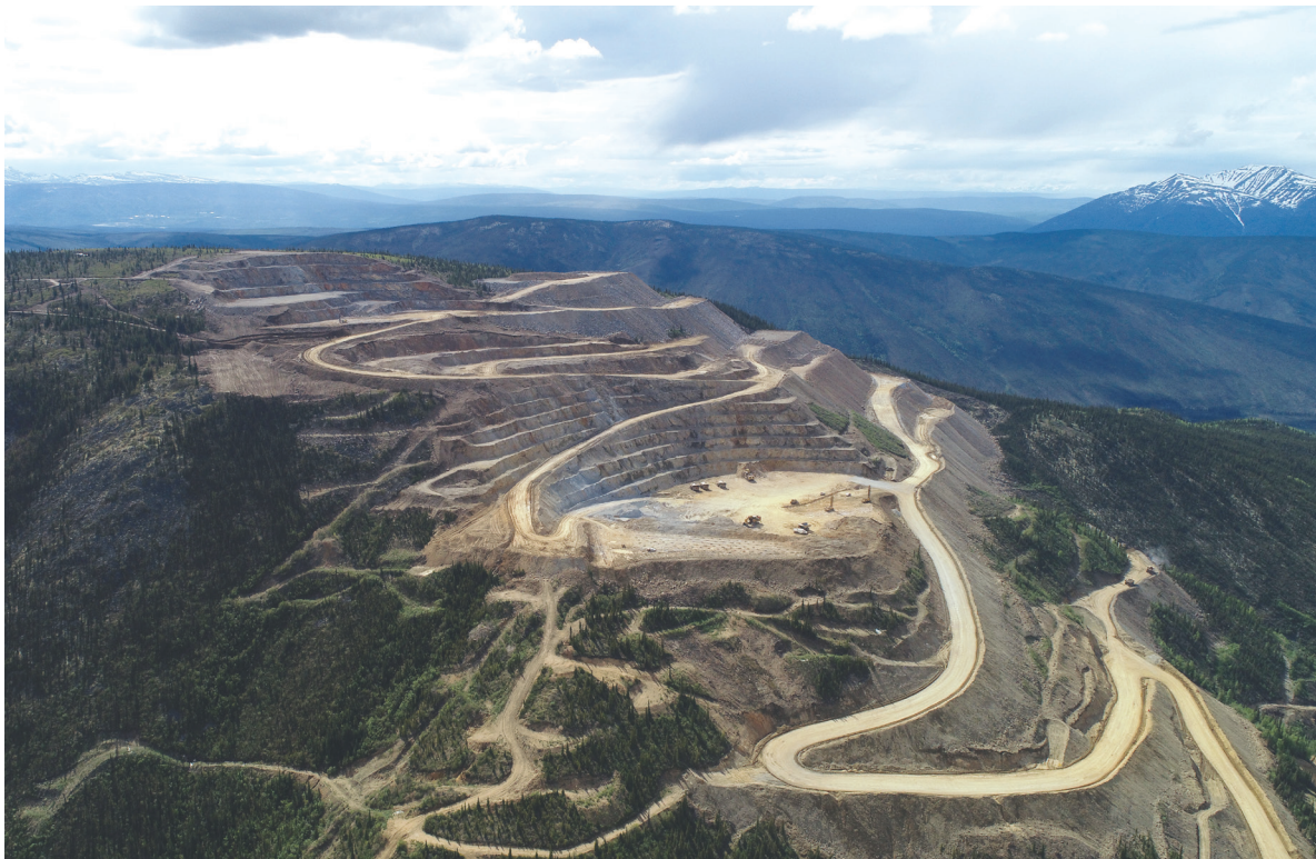
Aerial view of the Eagle Gold Mine open pit looking south.
